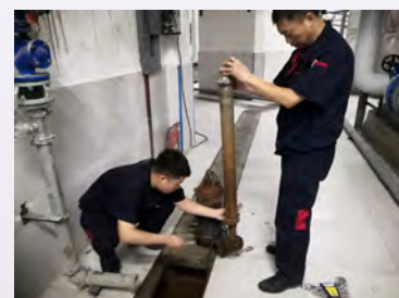
▲ Flood control inspection by Fang Xu during the heavy rain season
