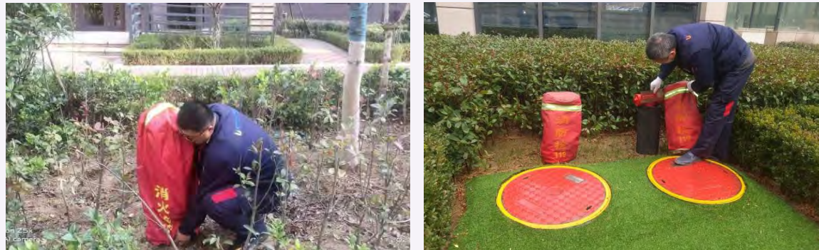
▲ The scene of outdoor cold insulation work
