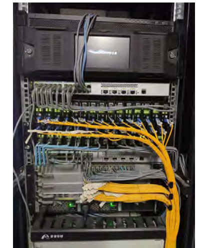
▲ Car park system inspection
