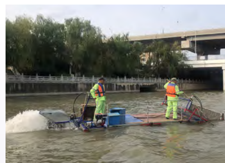
River Treatment for Xiaoqing River
